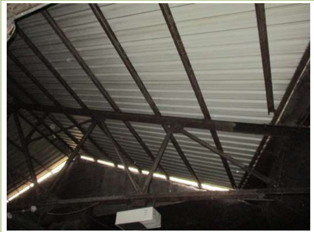
Metal roof cladding. No Asbestos Containing Materials (ACM's) detected
