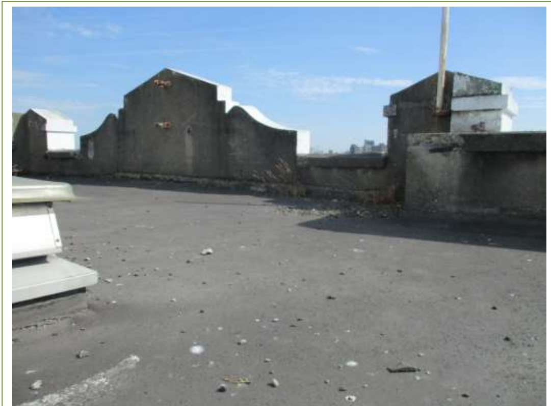
Asphalt on flat roof. No ACM's detected
