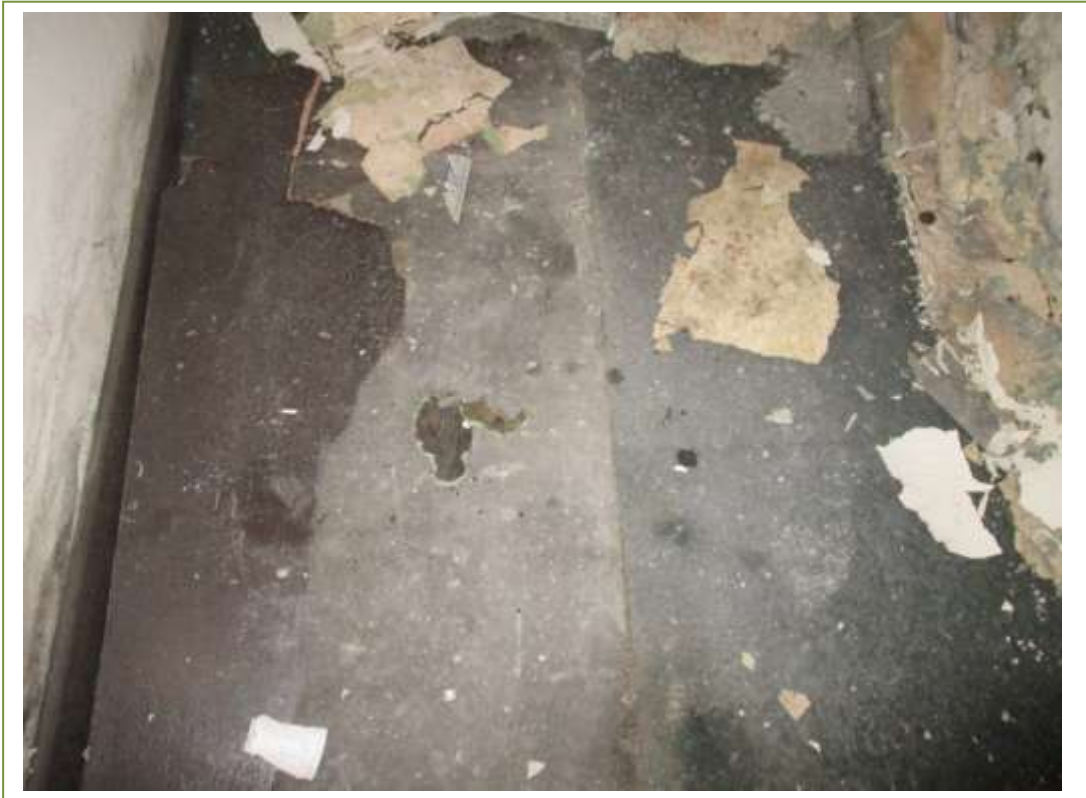
Floor coverings and asphalt in front areas. No ACM's detected
